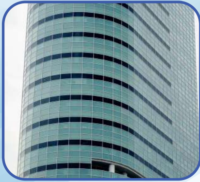
Pressure Boosting For Domestic Building And Comercial Building
