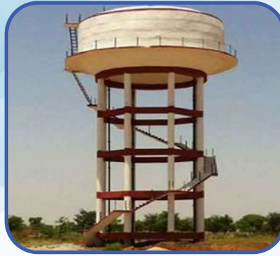
Water transfer from U.G to O.H Tank
